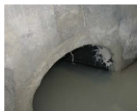
Example of a GOOD pipe installation. Pipe flush with the internal wall of the structure, clean grouting, and proper position.
