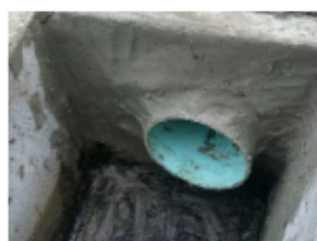
Example of a BAD pipe installation. Protruding past the internal wall of the structure, poor grouting, and wrong position.
